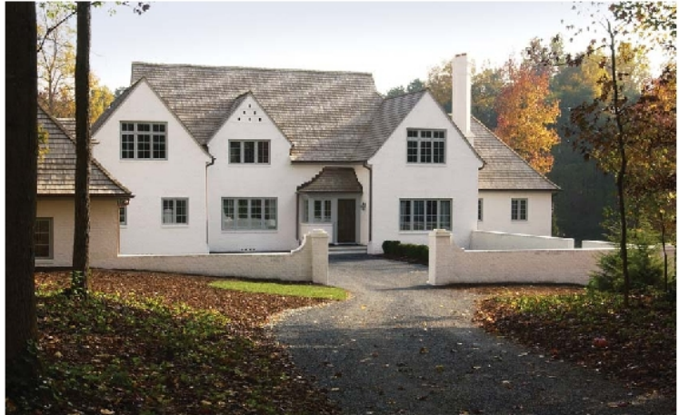
The entrance drive to James S. Collins' Fischer residence runs along the edge of the property and leads to a motor court of crushed granite, which provides off-street guest parking. A low garden wall screens the motor court to the west. The entry vestibule, sporting a bell-cast pine shingle roof with mitred hips, leads to the house's central hallway. All photos: Dennis Kale
