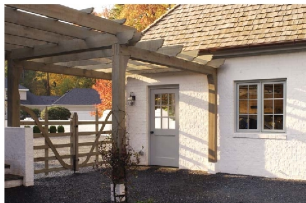
The garage is connected to the kitchen of the main house by a cypress pergola with a bleaching oil stain. Its columns and beams are mortise and tenoned with pegs and further strengthened with rabbeted shoulders. The outriggers with decorative cut ends are notched to the beam of the pergola. Note the gates that separate the motor court from the dog run. Diagonal yokes stabilize their mortise-and-tenoned and pegged stiles and rails.
